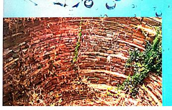
Abandoned well utilized for Ground Water recharging through rain water
